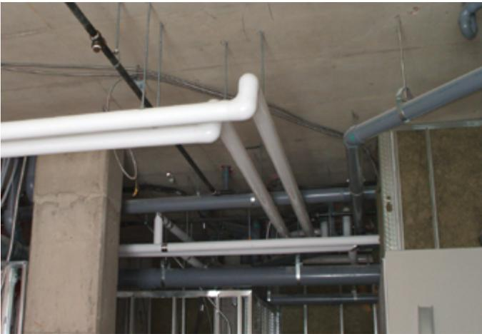
Made of time-proven CPVC, AquaRise delivers hot and cold potable water in commercial, industrial and high buildings. Its large inside diameter provides equal flow to copper and provides installers with competitive material costs and noticeable labour savings on the job site.
